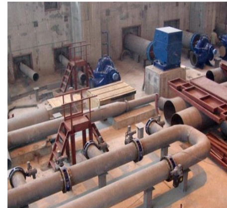
PUMPING STATIONS FLOORS
