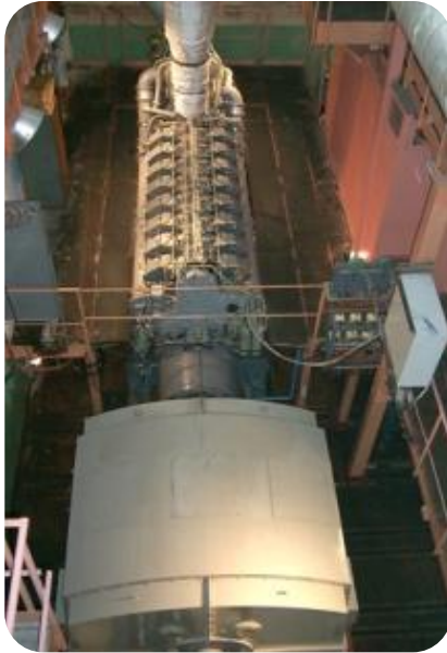
Genset for nuclear plant
